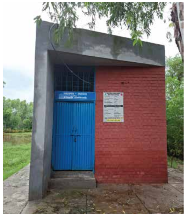
JJM Pump room in Ladana village in Ambala, Haryana
