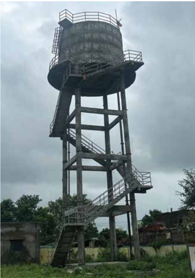
Water Tank built under JJM, Dewas
