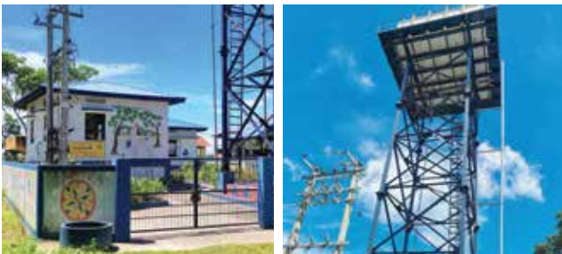
Water tank built under JJM in Sonitpur, Assam
