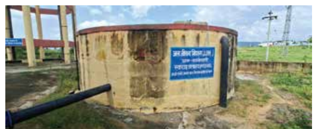
Water Tank built in Dausa, Rajasthan
